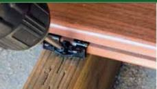
Fasten Deckmaster clips to the joist using the deck screws provided. Slide the screw into the deck clip guide hole and secure at a 45° angle into the joist.
