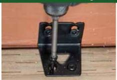
The first deck board needs to be fastened using angle brackets before using the clips. Use Deckmaster Hidden Deck Angle Brackets (HDA), item number DMACP. Fasten the HDA bracket to the bottom of the first deck board, then secure it to the header plate. Using the HDA bracket allows the first deck board to be fastened without screwing down through the top. Use Deckmaster clips once the first board has been installed.
